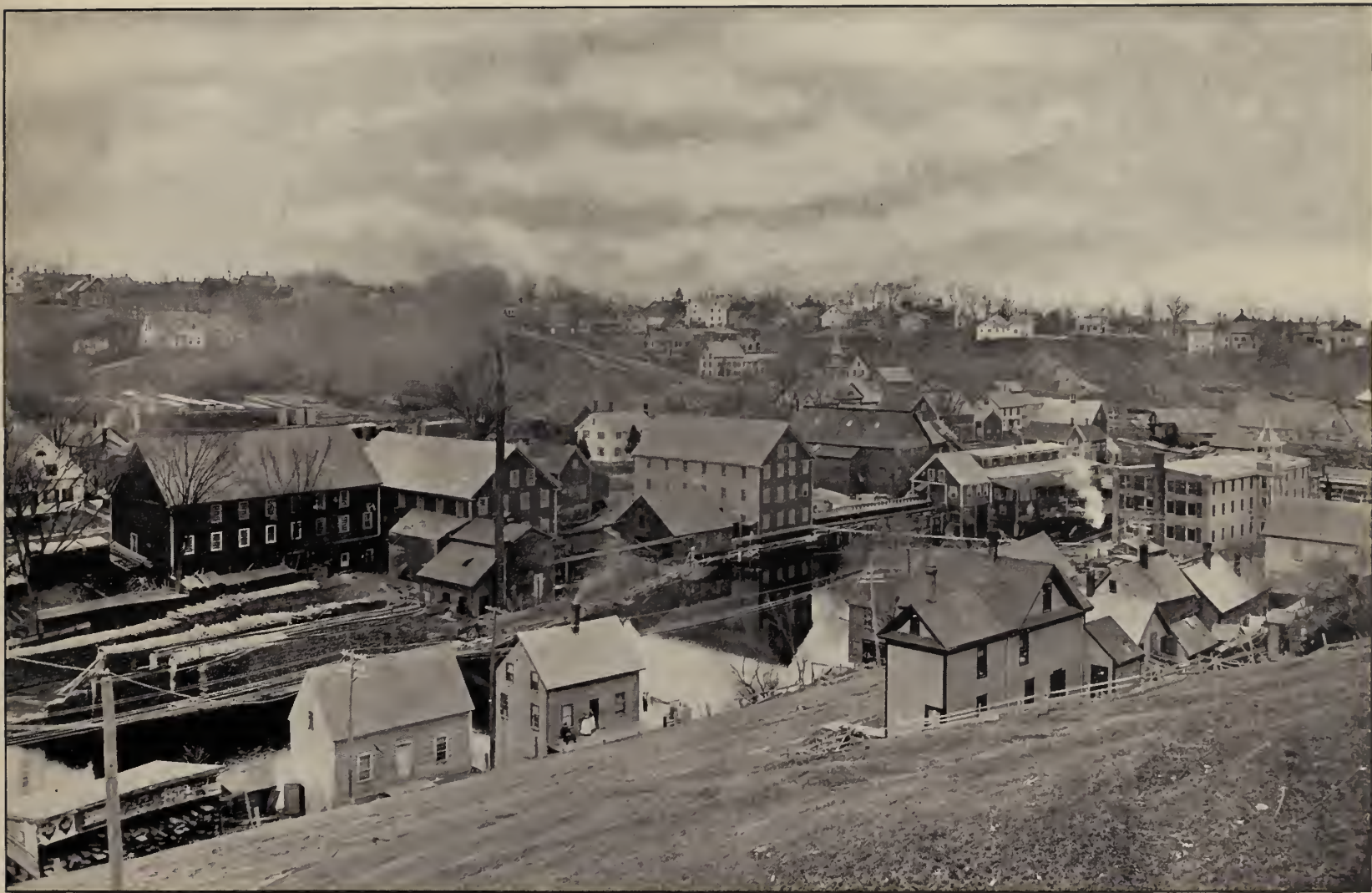
INDUSTRIES ON DAM NO. 2, FROM NEAL STREET.
